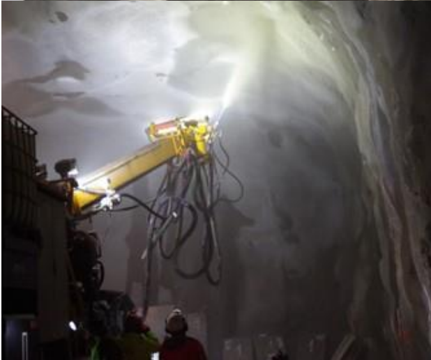
Fig. 10 Spraying of high-slump concrete, achieving exceptional immediate adhesion
