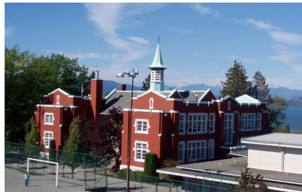
Bild 4: Queen Mary Elementary School, Vancouver
