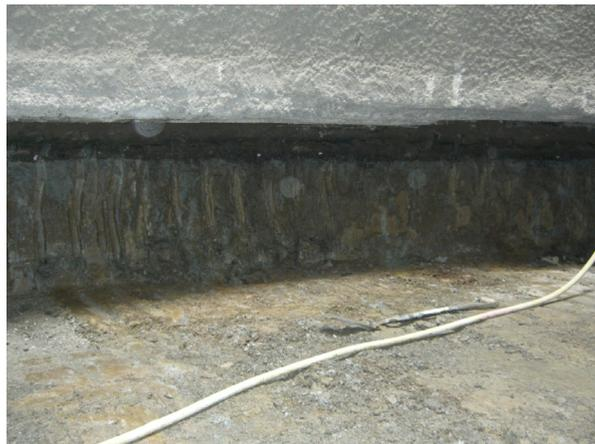
*Figure 11: Substrate prior to application on London Clay*
