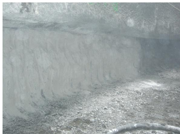
*Figure 12: Surface after application of TSL on London Clay*
