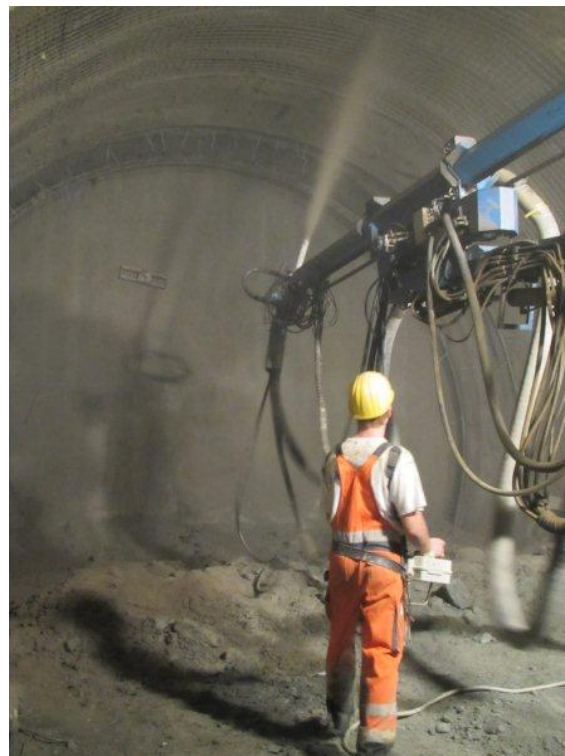
Figure 2: Spraying of mixture 6a
