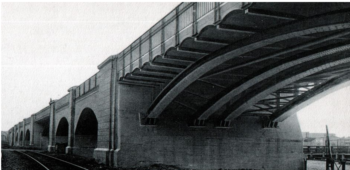
Figure 1. General view of the flyover with concrete and steel brick spans - Photo arch. 1914.
