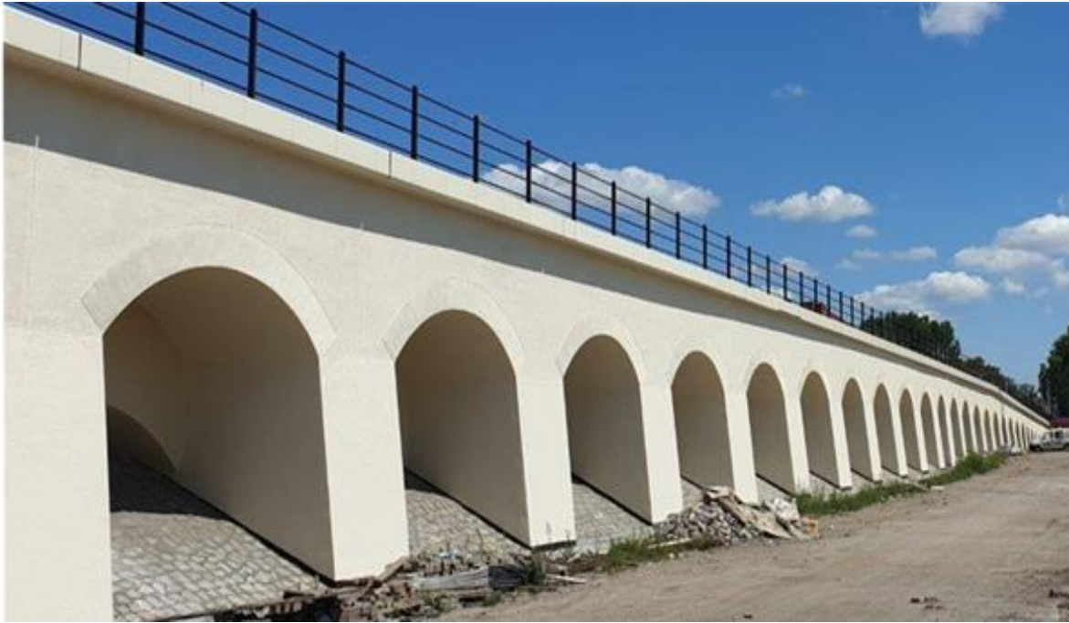
Figure 11: View of repaired flyover
