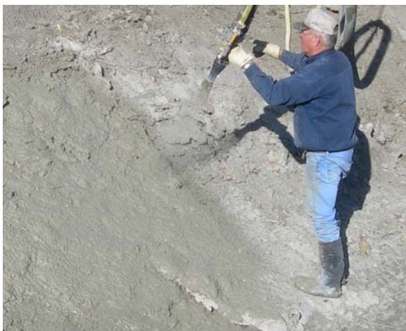
Figure 13: Irrigation channel lining installation using sprayed ECC in the western United States
