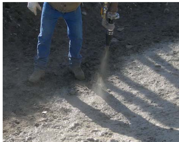
Figure 13: Irrigation channel lining installation using sprayed ECC in the western United States
