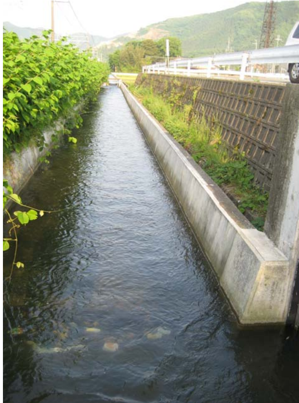
Figure 12: Irrigation channel repaired using sprayed ECC in Japan
